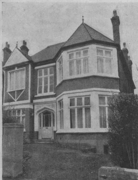
MUSLIM STUDENT CENTRE & HOSTEL, LONDON, UNDER RENOVATION
